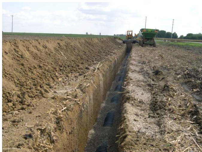
Figure 35: Subsurface drains being installed with a gravel envelope (from TG Drainage).
