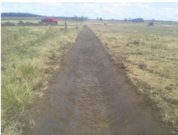
Figure 33: A freshly dug trapezoidal shallow spoon drain (DAFWA).
